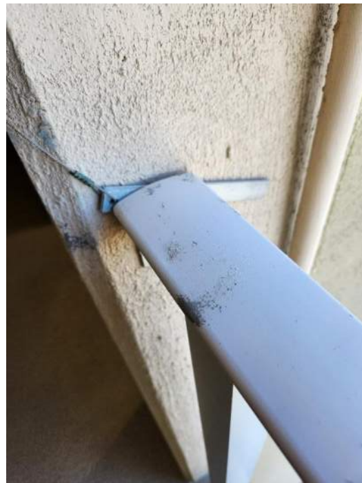
Photograph #12: Walkway Railing Coating
