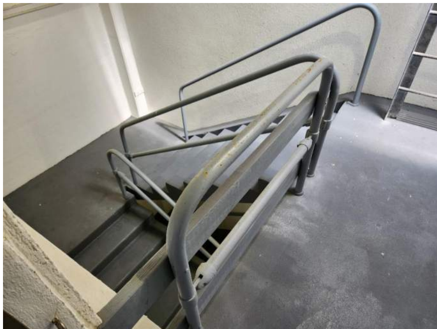
Photograph #10: Stair Railings
