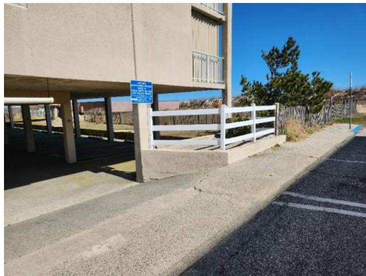
Photograph #6: South Entrance Ramp
