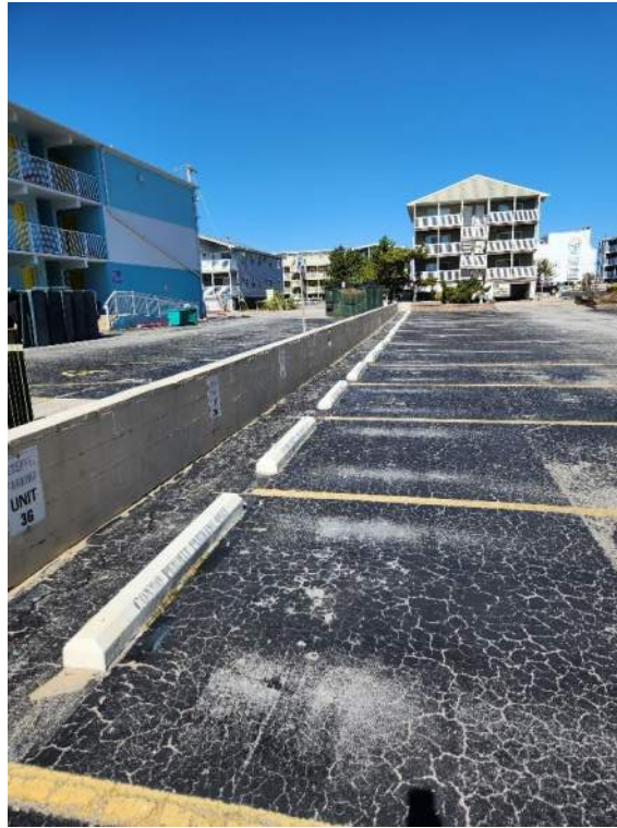
Photograph #5: Parking Area Landscaping Wall
