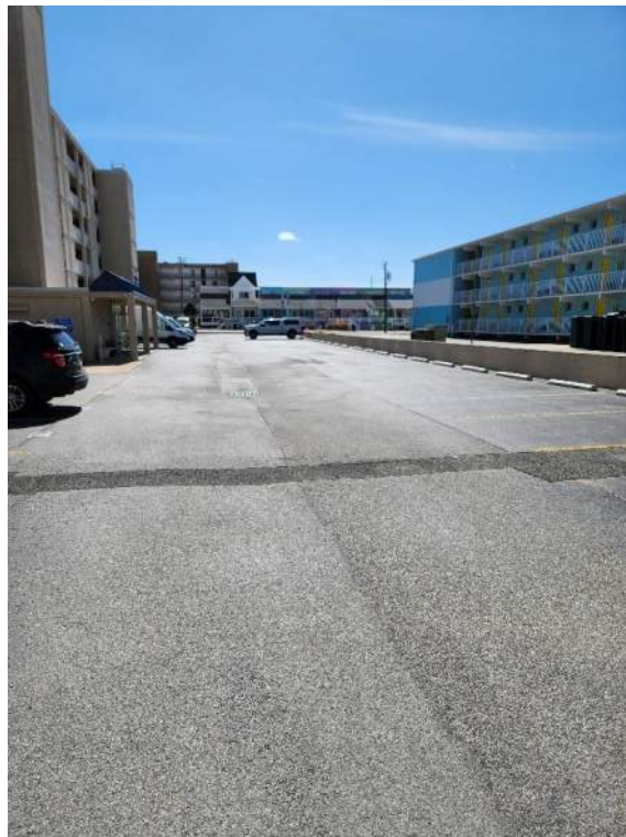
Photograph #2: Parking Area Asphalt
