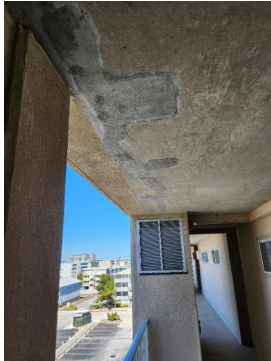
Photograph #11: Walkway Soffit Uncoated
