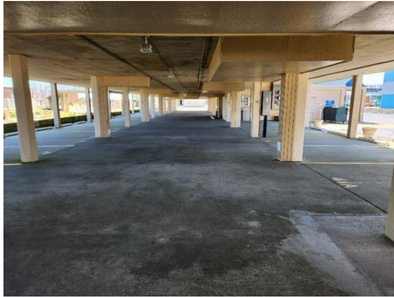
Photograph #3: Parking Area Under Structure
